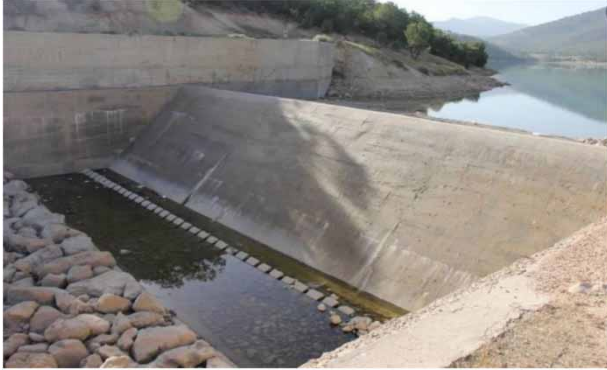
Figure 5 | An ogee spillway in a diversion dam in Iran.
