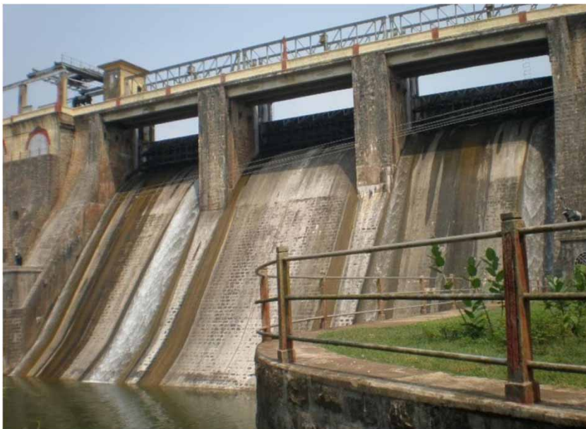
Figure 4 | An ogee spillway in Walayar reservoir, India.
