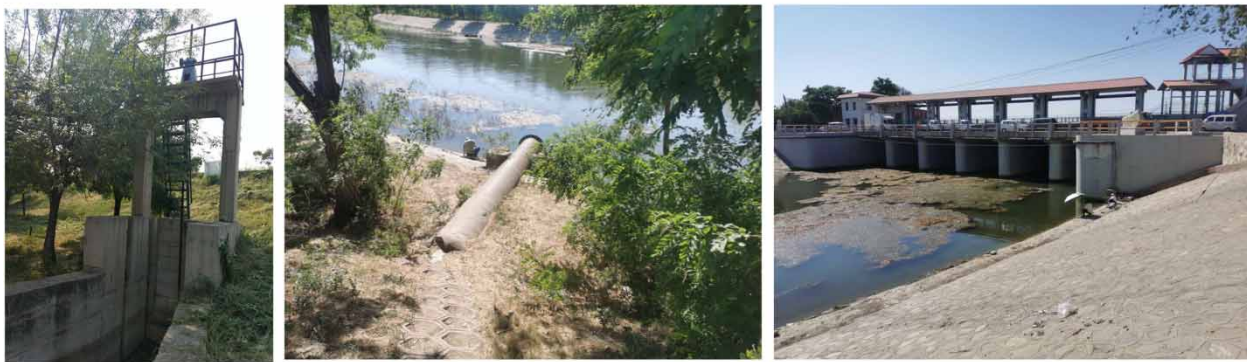
Figure 2 | Overview of the sewage outlet of the Duliujian River.
