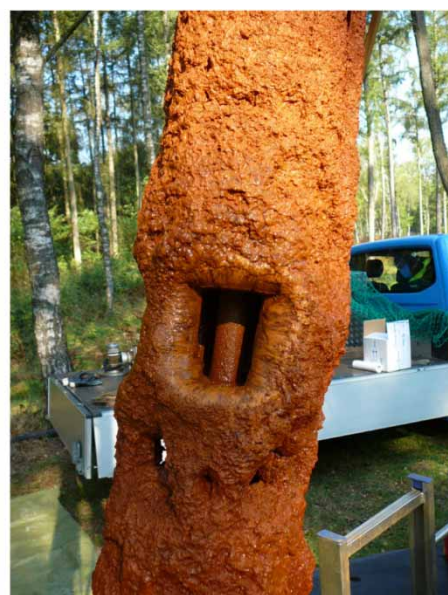
Figure 2 | Typical examples of iron oxide deposits in a riser pipe (125 mm diameter) and on a submersible pump of the Großenkneten well field after roughly six months of operation.
