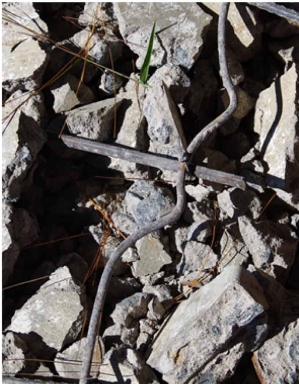
Figure 1 | Precast pit latrine flat slab. Top: reinforcement bar verification exercise. Bottom: reinforcement bar using recycled material.
