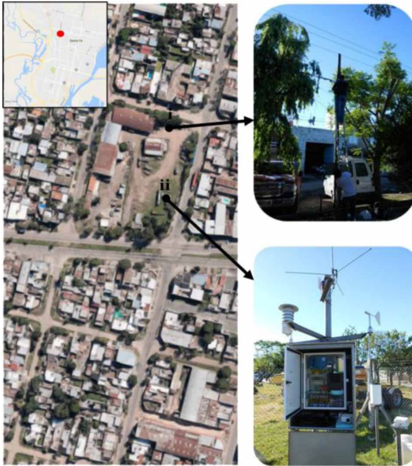
Figure 12 | Setting up the redundant transmission system on the Santa Fe station.
