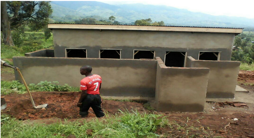
Figure 3.9 Example of in situ toilet/latrine construction by local mason: five stance lined pit latrine at Kisomoro Primary School, Uganda (Photo by Rutenta Allan, Source: https://rsr.akvo.org/fr/project/3890/update/19237 ).
