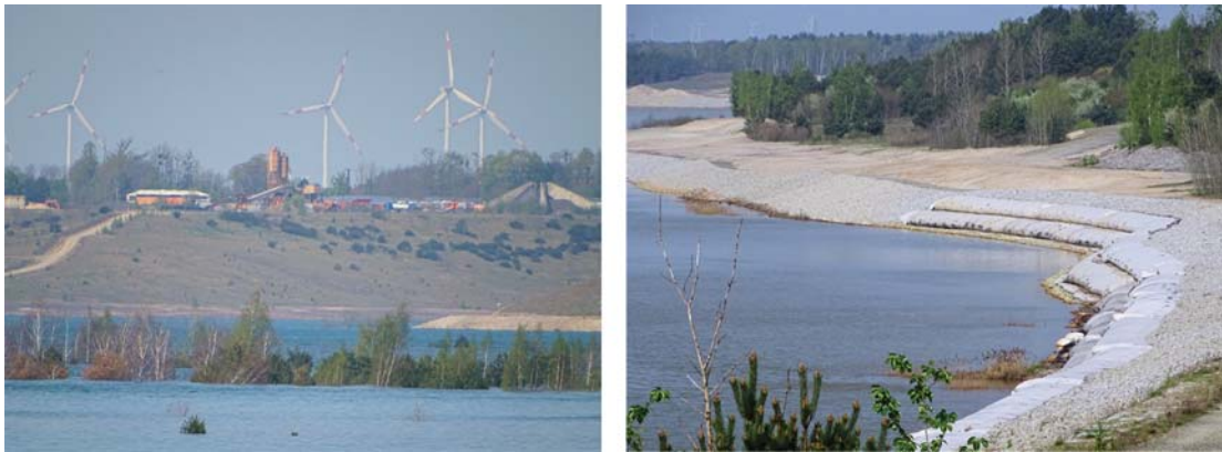
Figure 7.8 Example of a flooded open cast mine in the Lusatian area of Germany. The embankments are equipped with stabilising materials. (Photographs: Petra Schneider )
