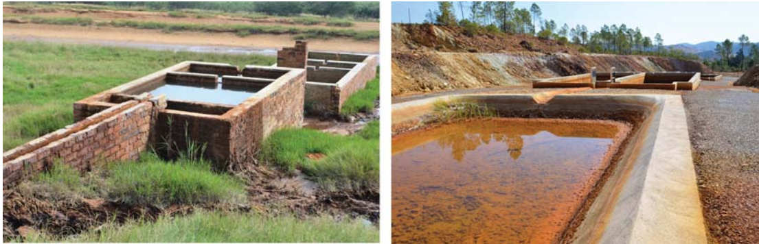
Figure 7.12 Example of a passive mine water treatment system in South Africa (left), and the Río Tinto area, Spain (right). (Photographs: Petra Schneider )
