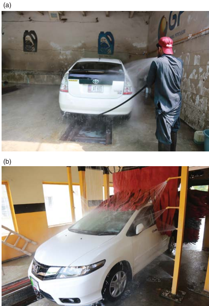
Figure 11.6 (a) A conventional car wash without water recycling and (b) modern car wash with altered nozzle and water recycling. Peshawar, KP Pakistan. (Credit: Tahir Saleem, 2019).
