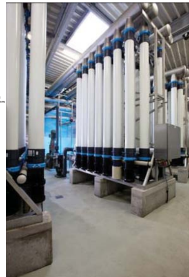
Figure 8.3 In 2010, the city's wastewater treatment plant was equipped with a membrane bioreactor (owned by Evides), which increased the treatment capacity of the municipal plant by 20% and dramatically improved the quality of the effluent (called permeate) sent to Evides' reverse osmosis treatment facility for the production of demin water. (Credit: Evides Industriewater, Rotterdam, the Netherlands)
