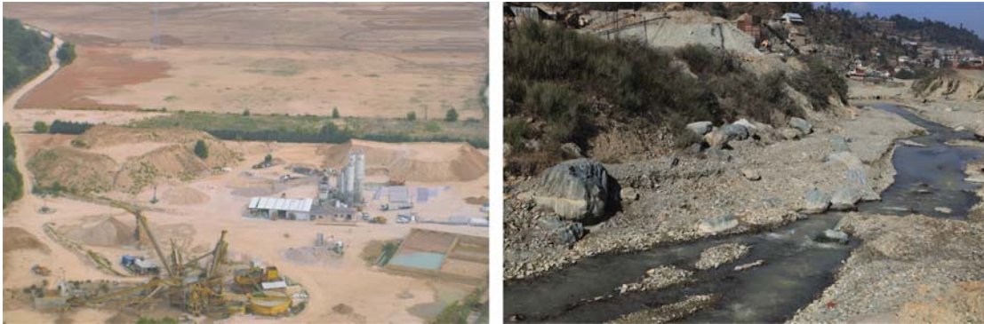
Figure 7.6 Example of an aggregates mine and the respective extraction and processing installations in the Sevilla region, Spain (left) and increased sedimentation due to aggregates mining in the Naku Khola River, Kathmandu Valley, Nepal. (Photographs: left, Petra Schneider; right, Christian Wolkersdorfer )
