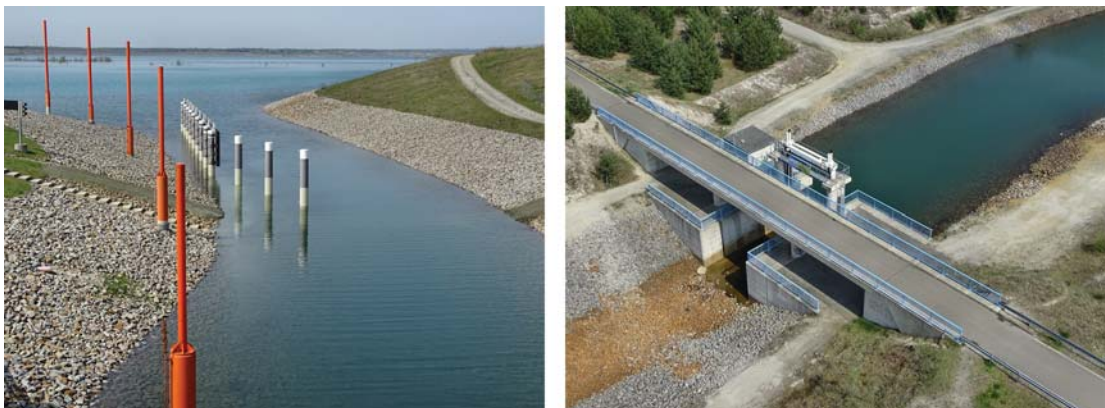
Figure 7.10 Flooding water channels for transport of water during the rehabilitation process. After rehabilitation, these channels serve as waterway for small touristic boats. (Photographs: Petra Schneider )
