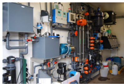
Remote control, online monitoring (P, F, T, pH, NTU)
