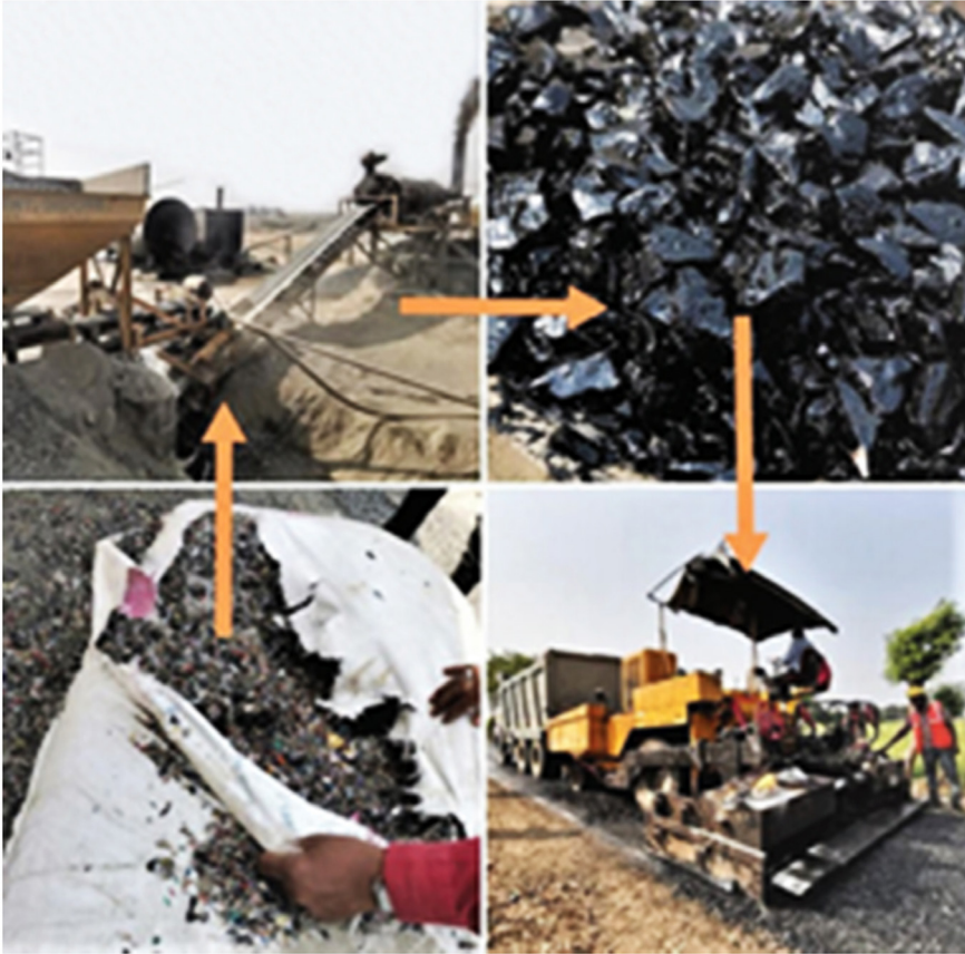
Figure 6.58 Incorporating PW into a road asphalt mixture using the dry process (Source: Heriawan, 2020 ).
