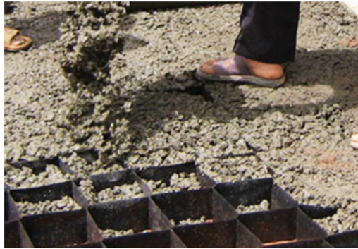
Figure 6.59 Plastic cells filled with cement concrete (Source: Heriawan, 2020).
