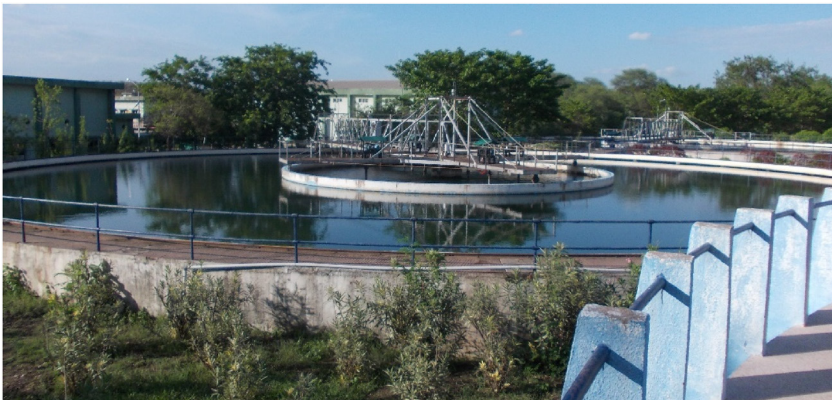
Figure 2.9 Flocculation chamber in water treatment plant (courtesy of Nagpur Municipal Corporation and Orange City Water Private Limited, Nagpur, India).
