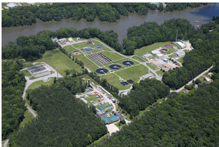
Figure 7.4 The Hampton Roads Sanitation District (HRSD) York River Treatment Plant (YRTP) in Seaford, VA.
