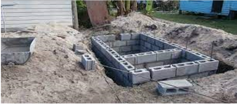
Figure 3.8 In-situ block work septic tank by local mason (Source: https://niwa.co.nz ).
