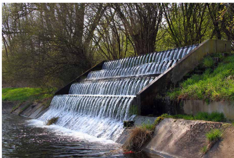
Figure 1 | Low-cost cascade aeration system that enhances the air–water transfer of atmospheric gases (e.g., oxygen and nitrogen) and volatile organic compounds. The term ‘green technology’ commonly invokes images of such technologies; however, green technologies span a broad spectrum of treatment typologies.
